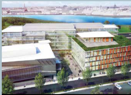
5. CURTIS PROPERTIES AT MLK & W
