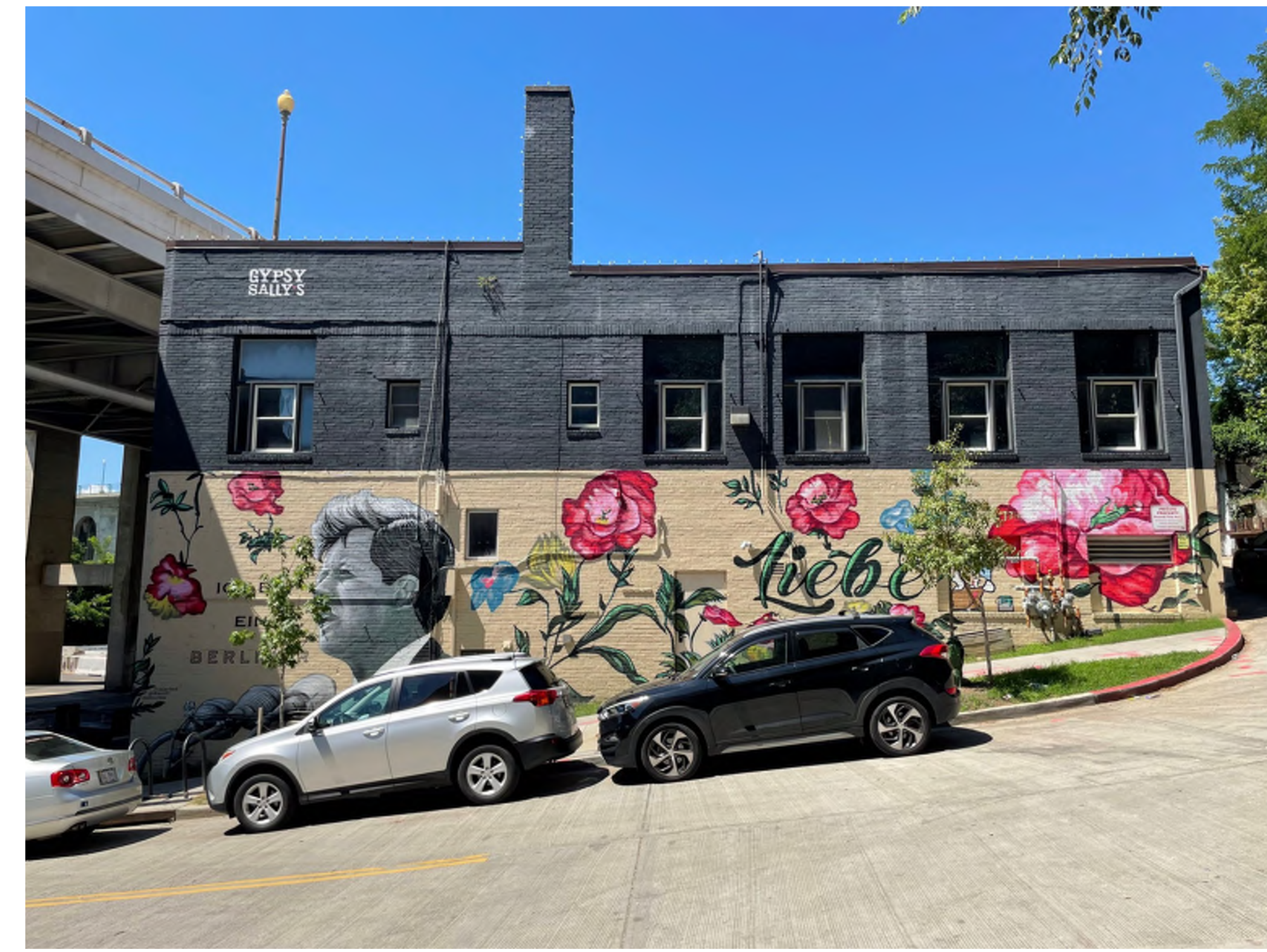
EXTERIOR - EXISTING EAST ELEVATION (34TH STREET)
