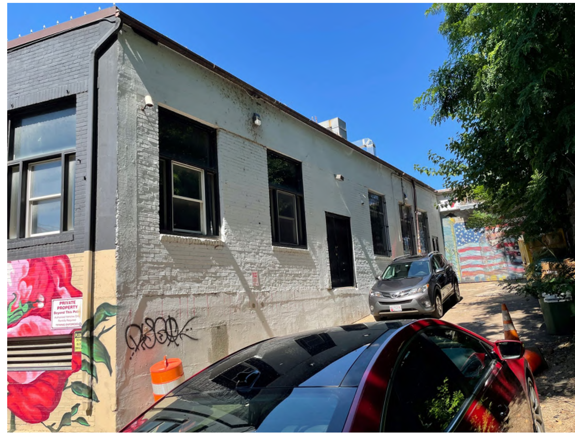
EXTERIOR - EXISTING NORTH ELEVATION (LOADING DOCK)
