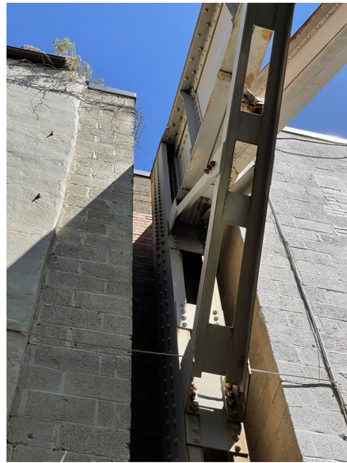
EXTERIOR - SOUTH ELEVATION (WHITEHURST FREEWAY SUPPORT)
