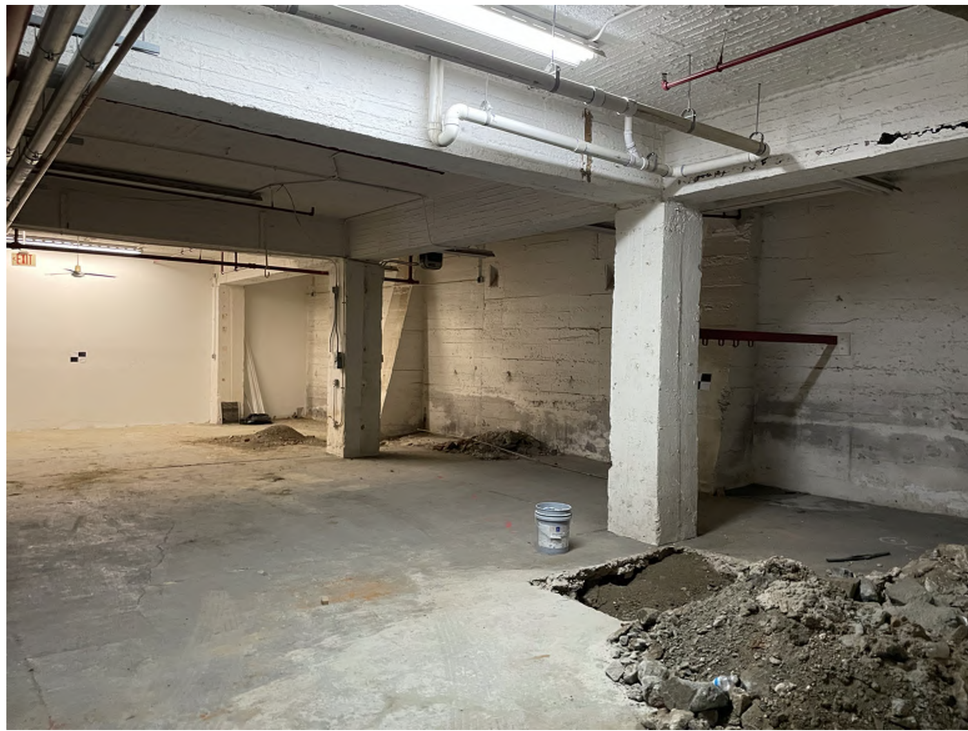
INTERIOR - EXISTING 1ST FLOOR VACANT SPACE
