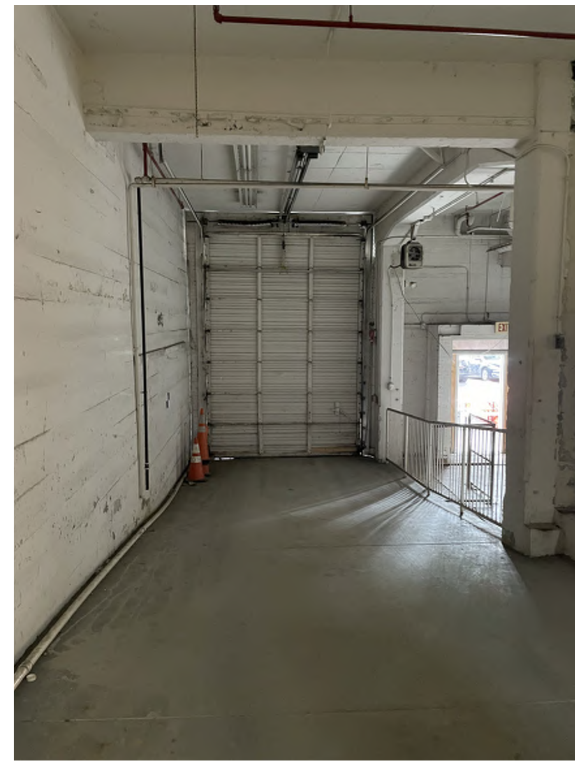
INTERIOR - EXISTING 1ST FLOOR LOADING
