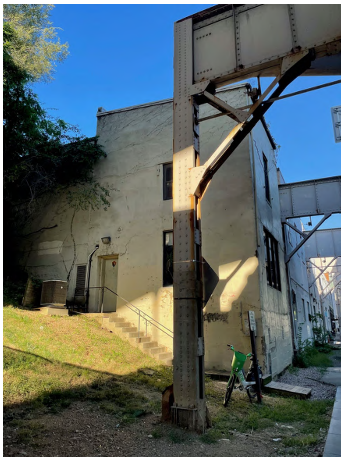
EXTERIOR - EXISTING WEST ELEVATION (KEY BRIDGE)
