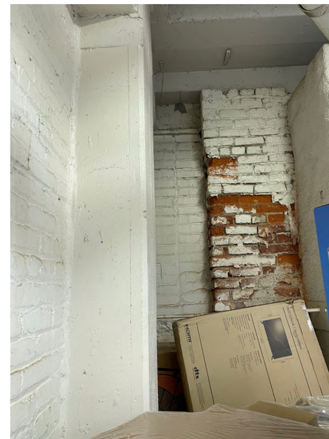
INTERIOR - EXISTING BRICK
