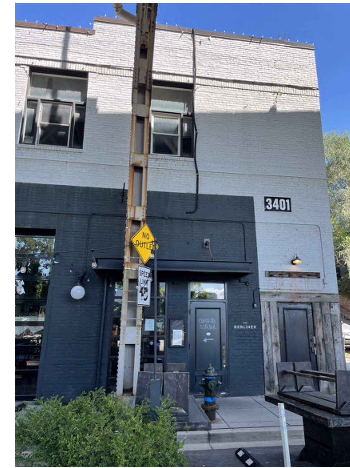
EXTERIOR - EXISTING SOUTH ELEVATION ENTRY DOORS
