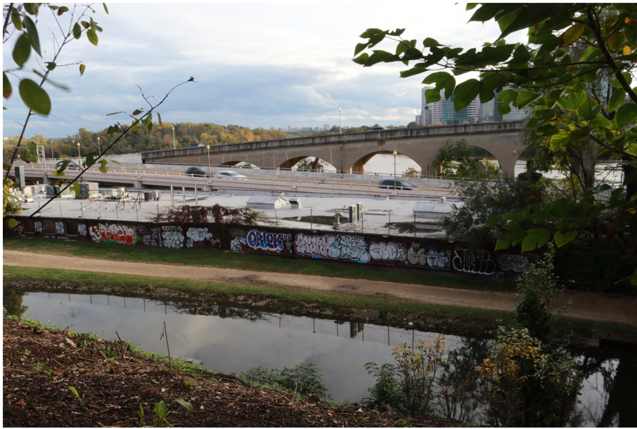
EXTERIOR - EXISTING NORTH ELEVATION (CANAL SIDE) & ROOF
